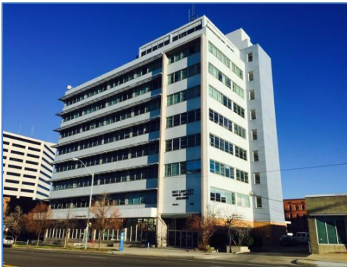
Pacific Northwestern Pipe Building
