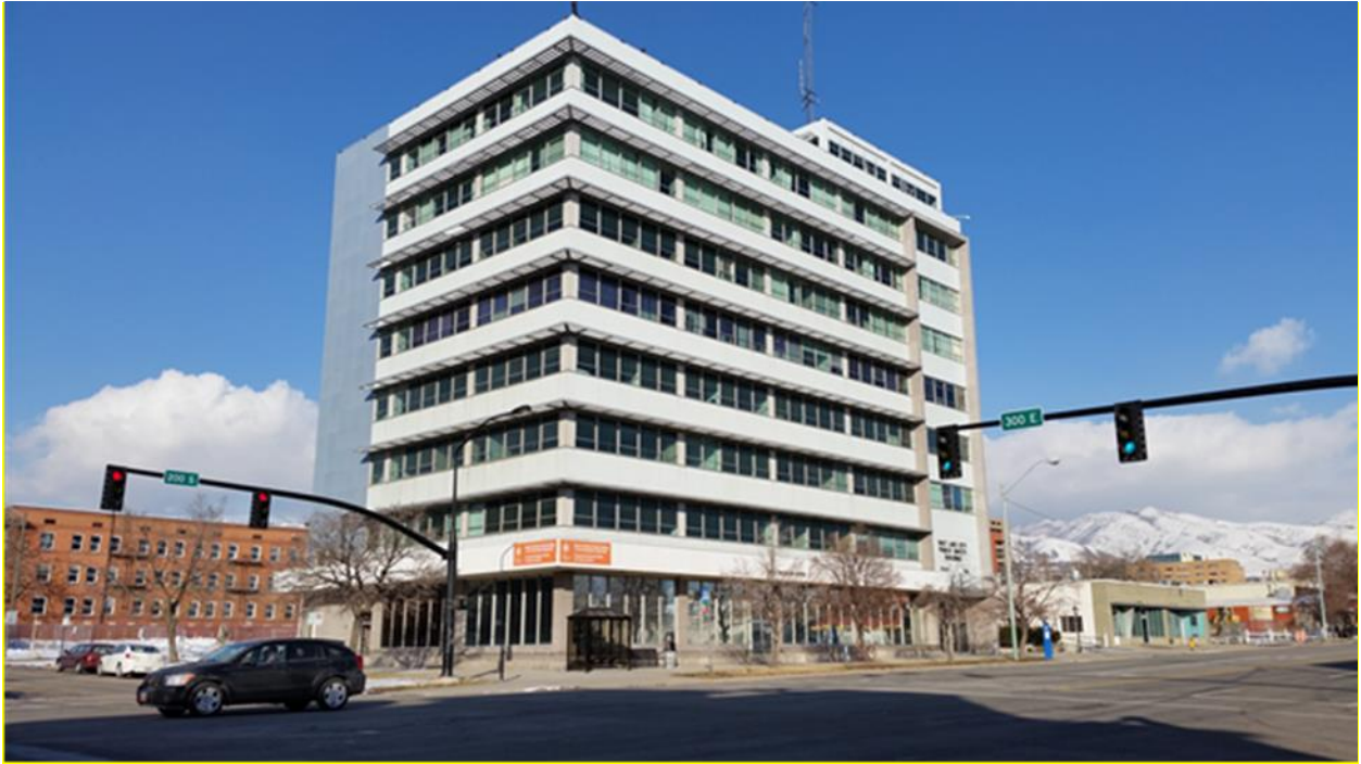
Main structure to be restored
